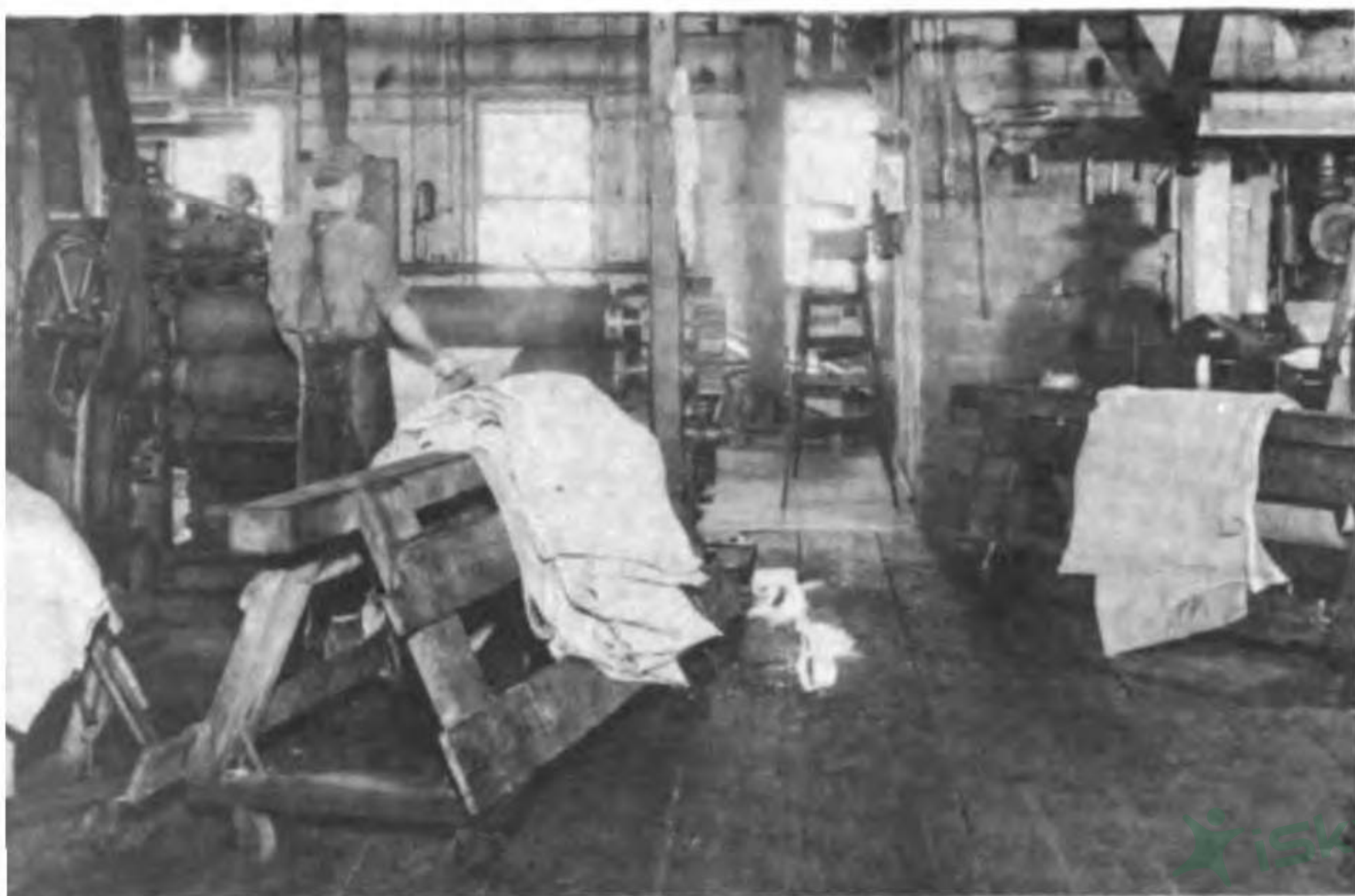
202. The Leather Press Removes Excess Moisture from the Hide after Tanning
