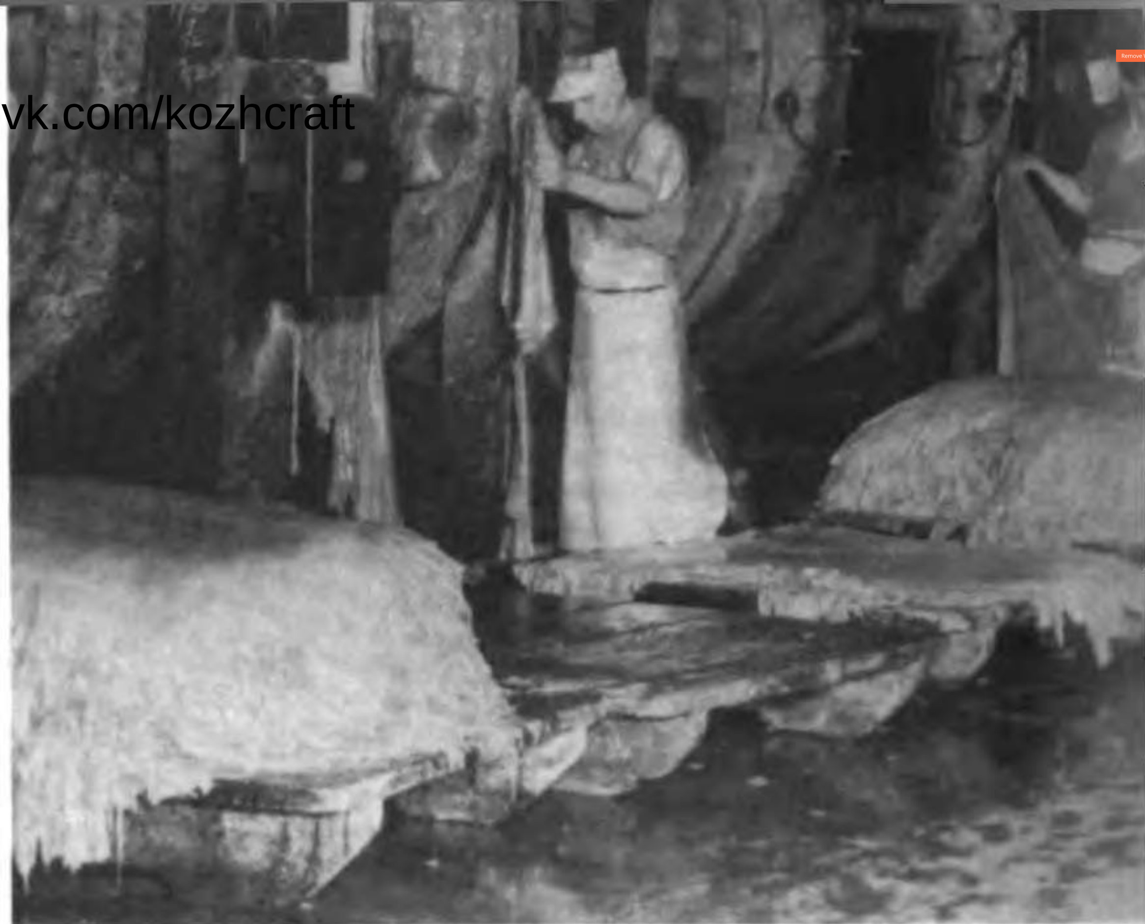
204. Skins and Hides Being Removed from the Chrome Tanning Drums
