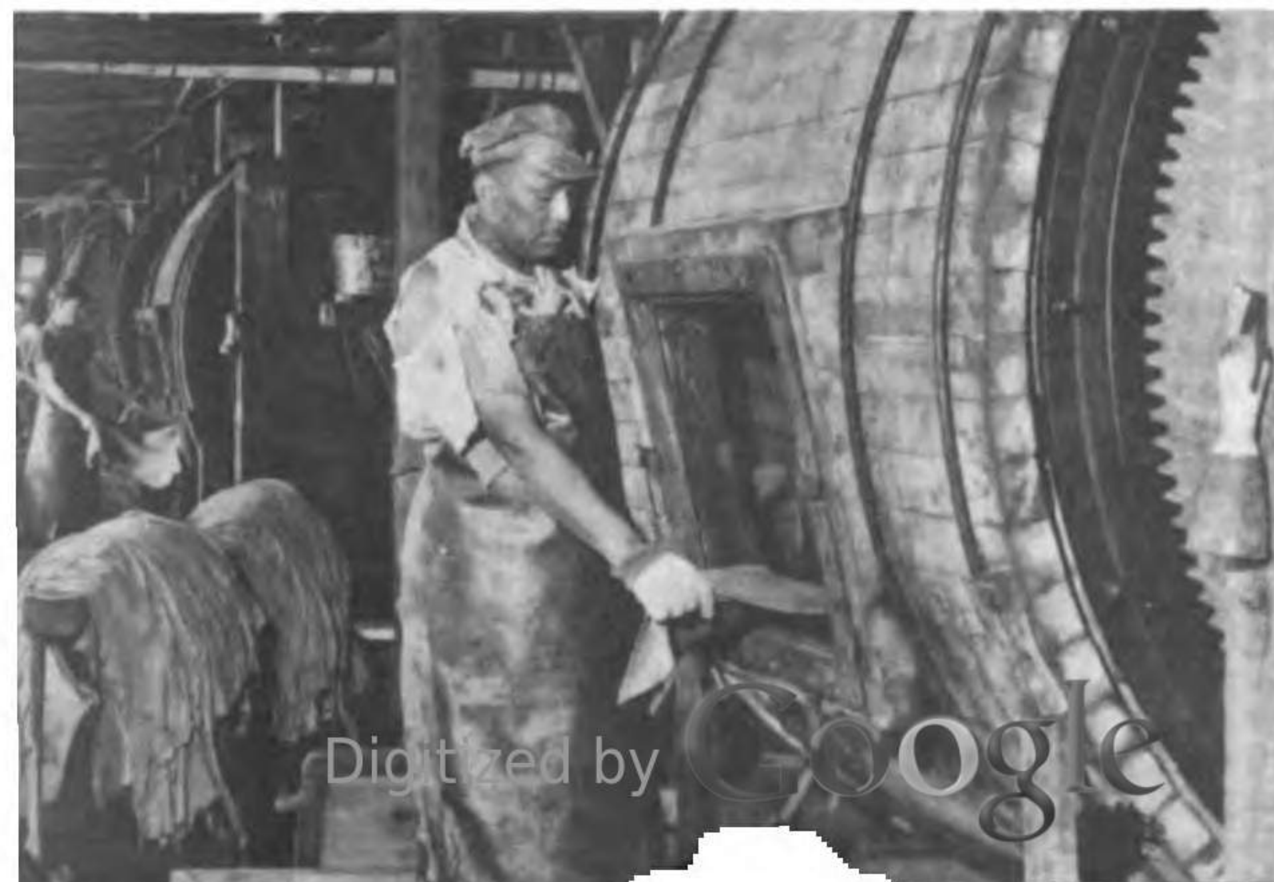
203. Skins and Hides Being Put into Mechanical Drums to Be Treated with Oil and Greases
