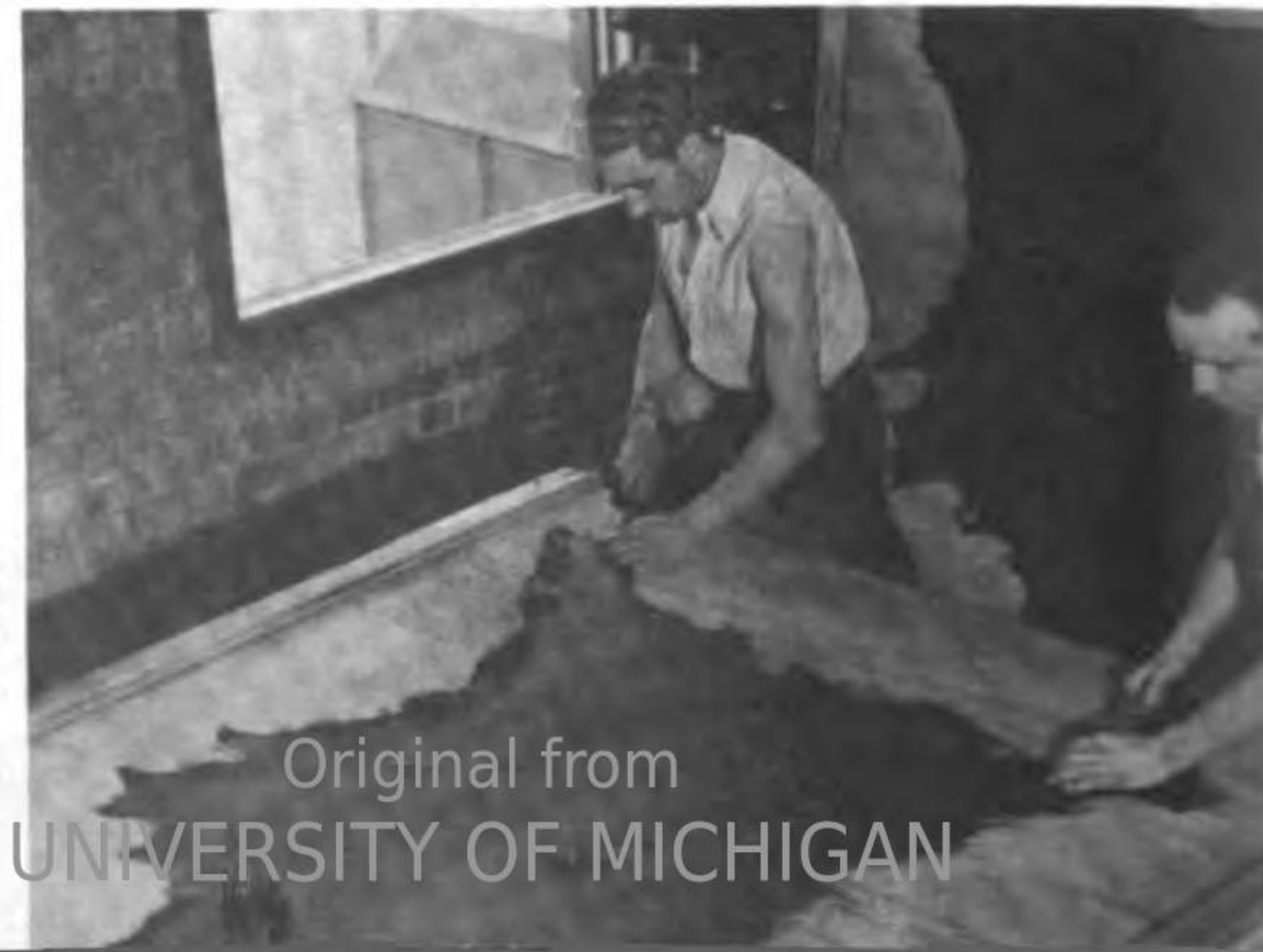
206. Skins and Hides Must Be Tacked on Frames So They Will Not Wrinkle in the Oiling and Coloring Process
